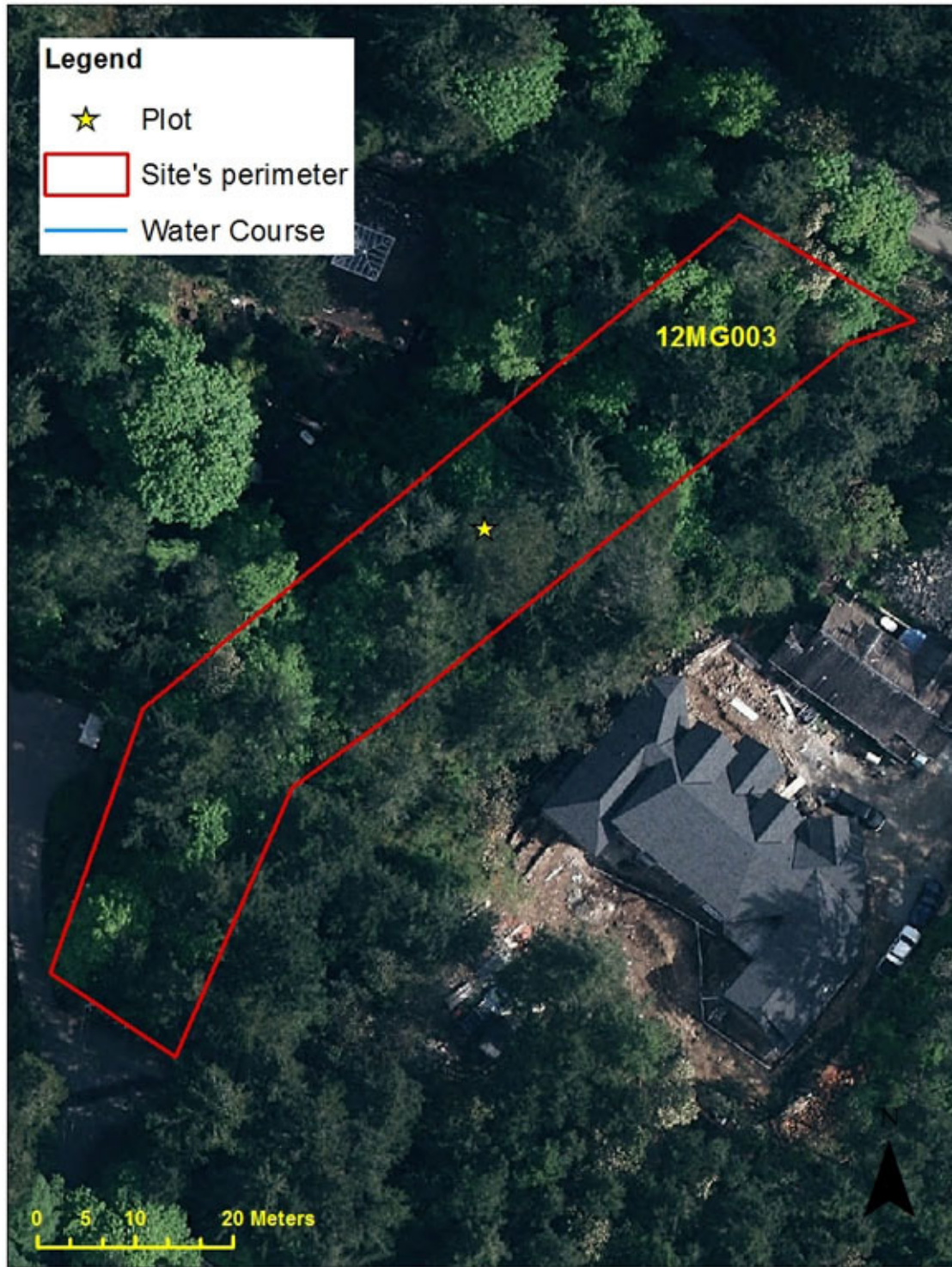
FIGURE 3 Site 12MG003 – Undeveloped Right-of-Way Sherwood Dr.
